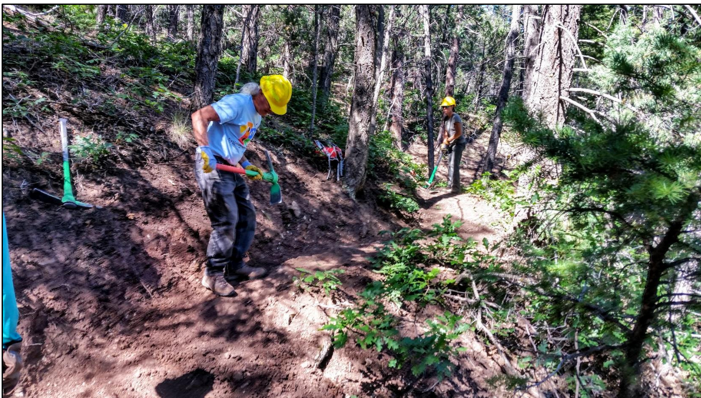
Coming out of the turn, we dealt with the usual roots, backslope, rocks, and tread leveling.
