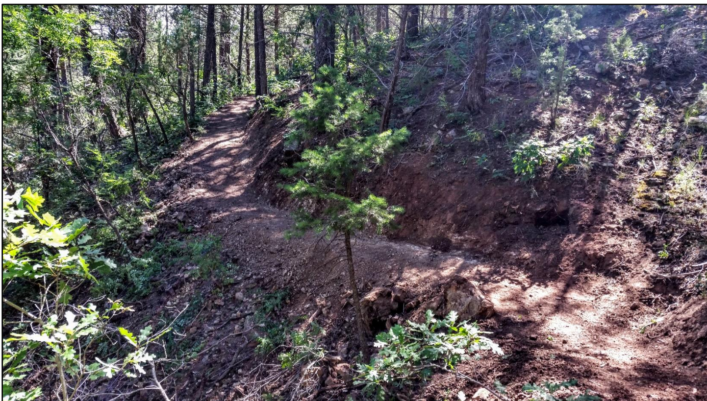
Finished turn on TC06. Quite a bit of this section has very steep sideslope.
