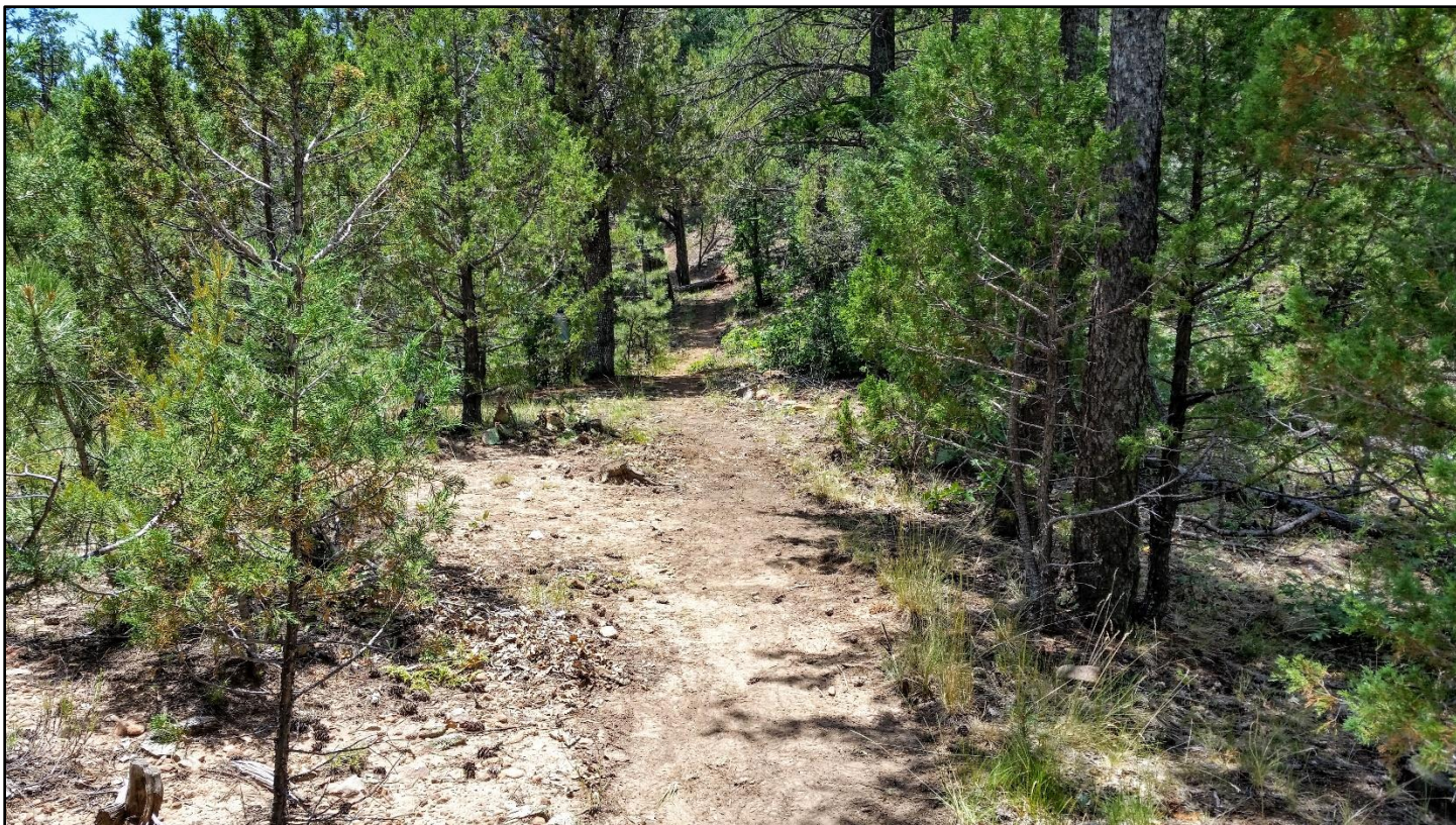
Connection completed. Next session the crew will work on up towards Faulty Trail.
