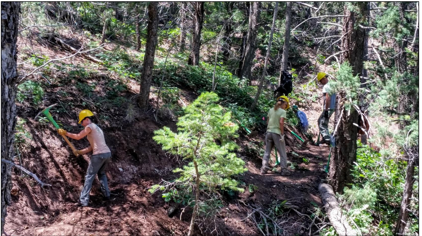
We're talking VERY steep backslope to cut back on this section.
