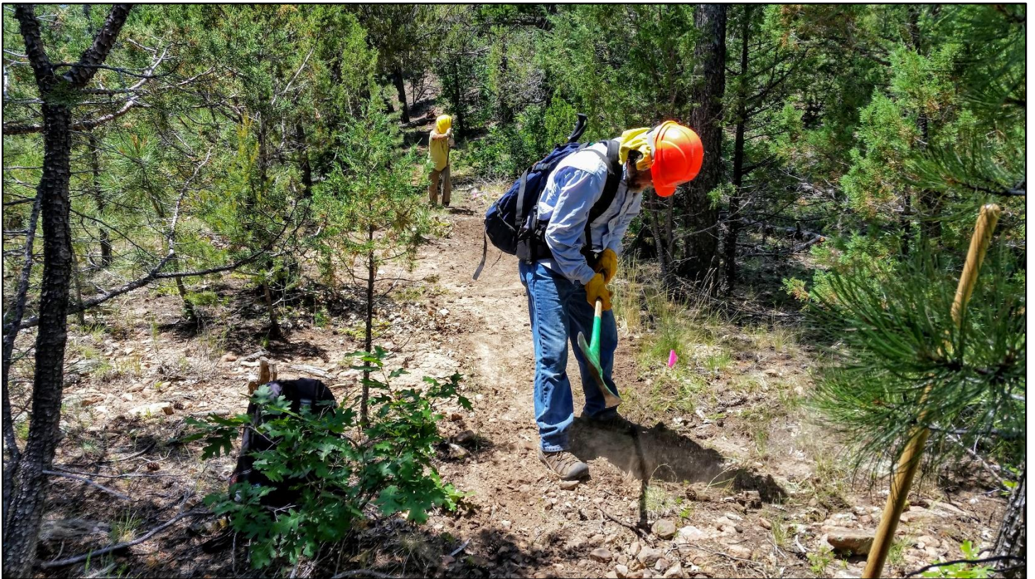
And the tread had to be cut in. It is very satisfying completing a long section.
