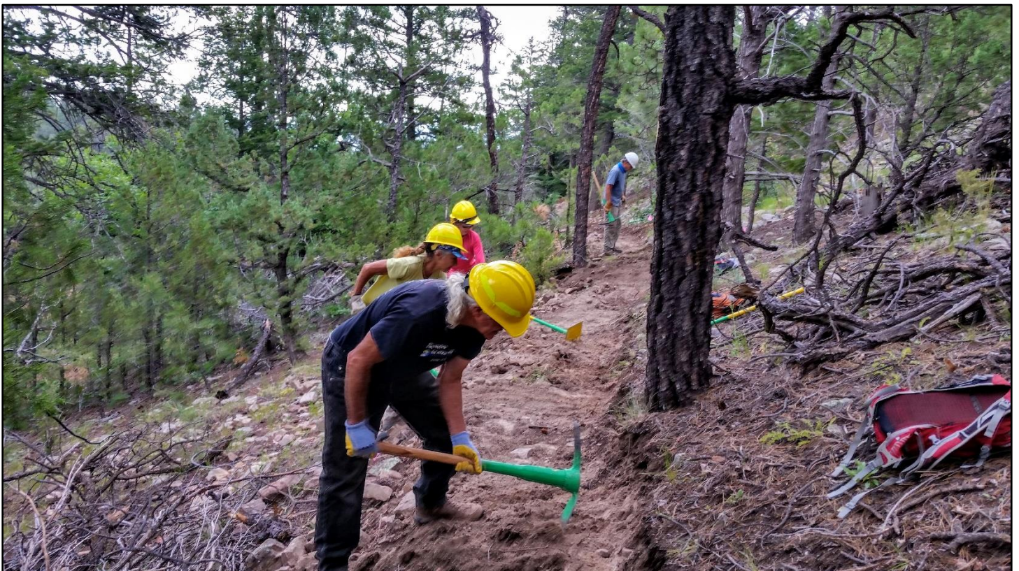
Many rocks and very fine soil. But the crew starts to make tread appear.
