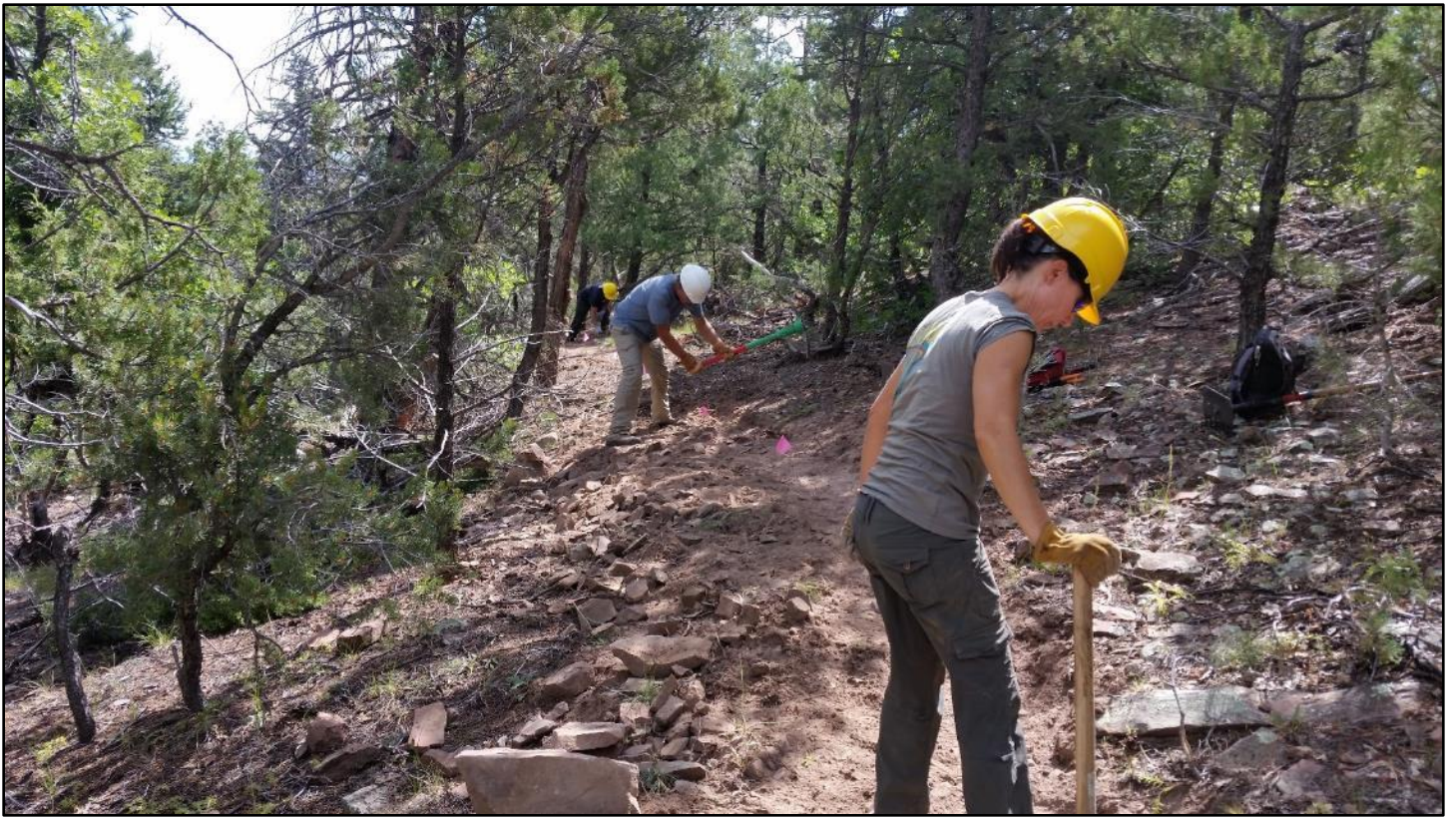
Further down the crew still fought rocks, rocks, and more rocks.
