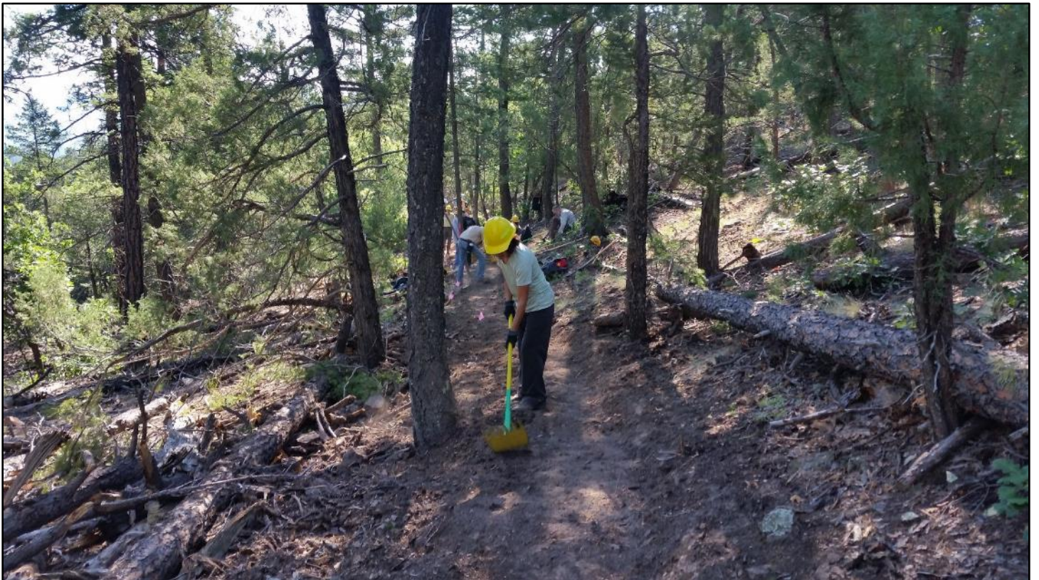
A careful trail finisher grooms the tread after the line is hogged out.
