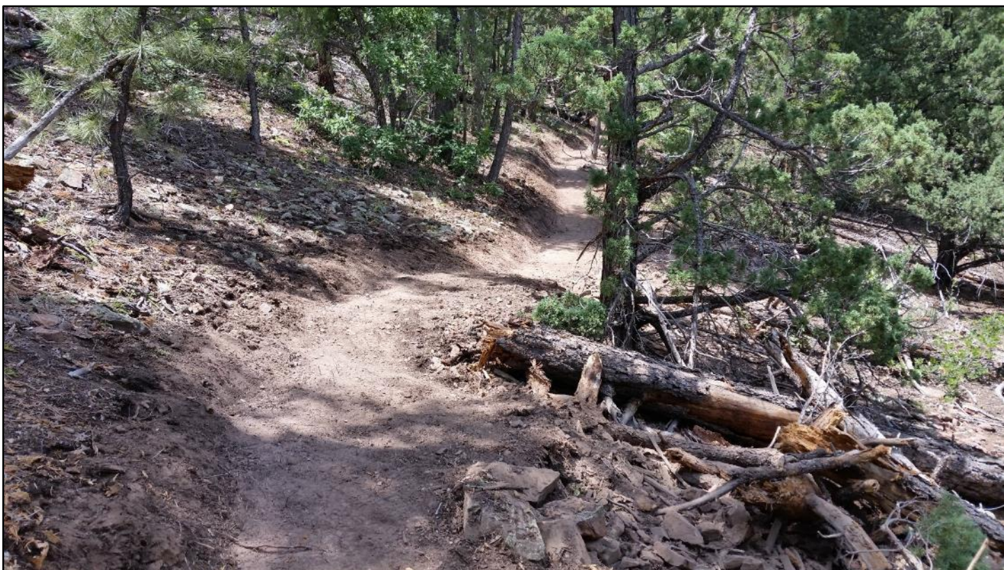
Good trail design includes grade reversals and undulation. This section came out very nice.
