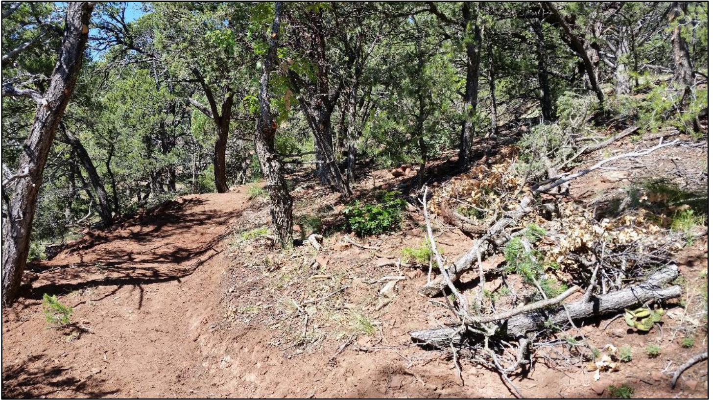
After: the steep section is obliterated, replaced by a more sustainable turn.
