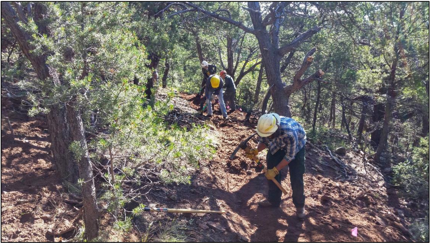
The boss makes final adjustments to the new bermed turn.
