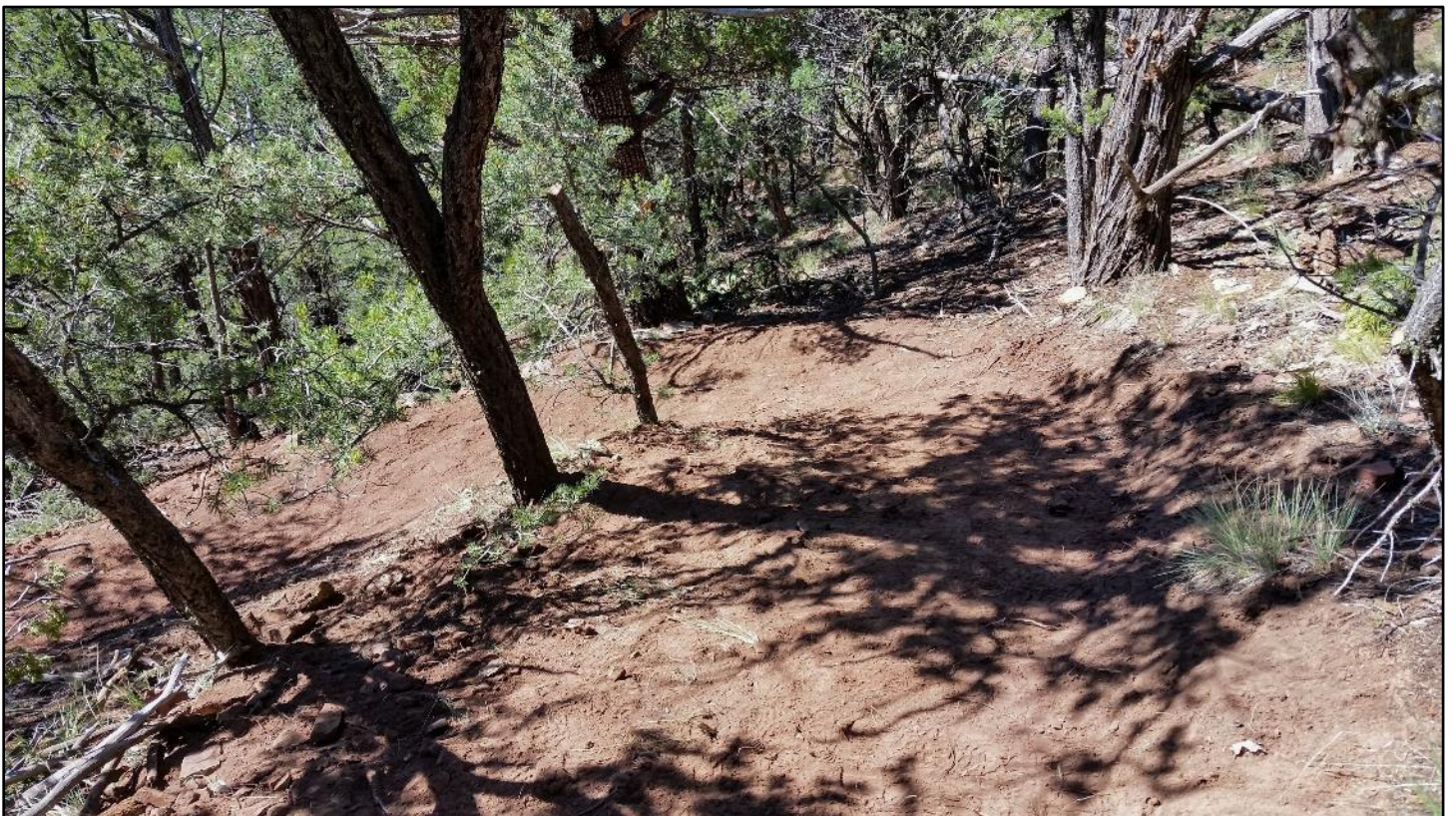
The nice sustainable bermed turn is complete.
