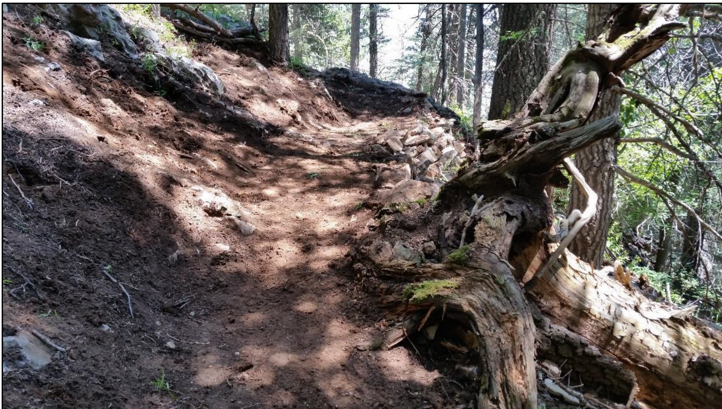
Boom! Finished tread on the cribbed section: the FOSM trail crew just loves this stuff.
