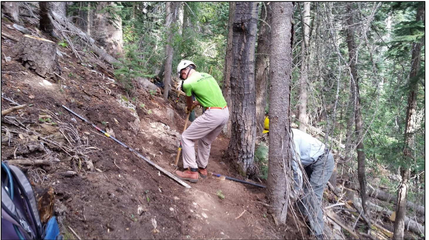
The Boulder Boys coax a limestone slab out of a tight section of trail.
