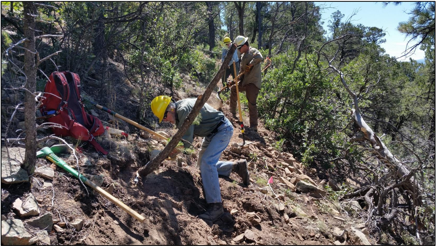
Low-stumping a small pinon. Luckily this one did not need to be dug out.
