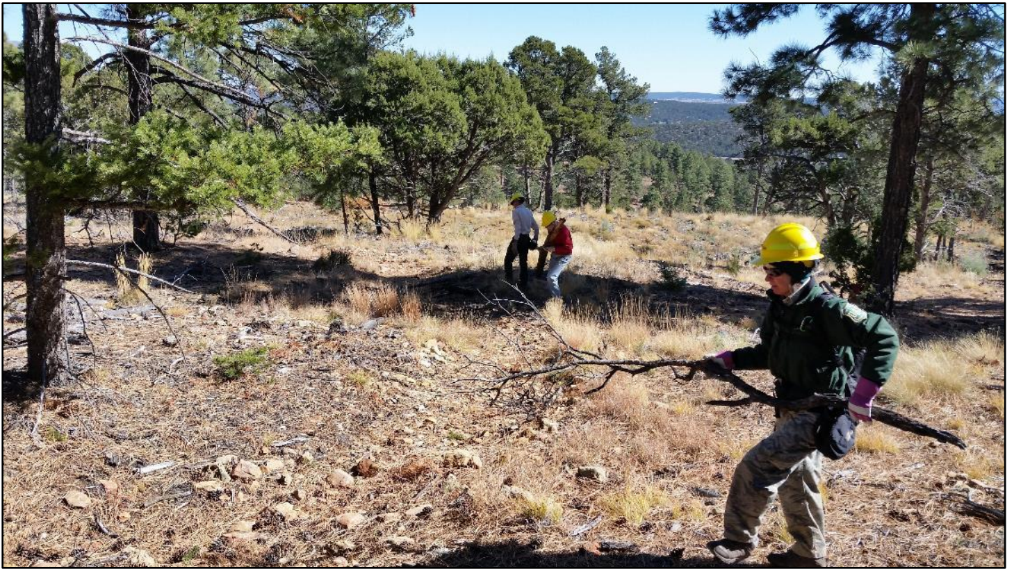
After lunch, the crew worked to complete obliteration of the old user trail bypassed by Madera Locura.
