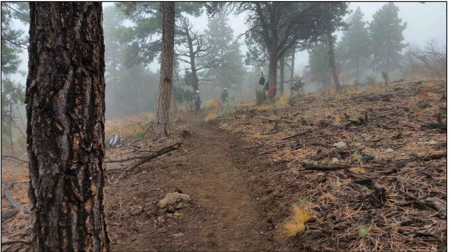
After: The crew moves on to the next section.
