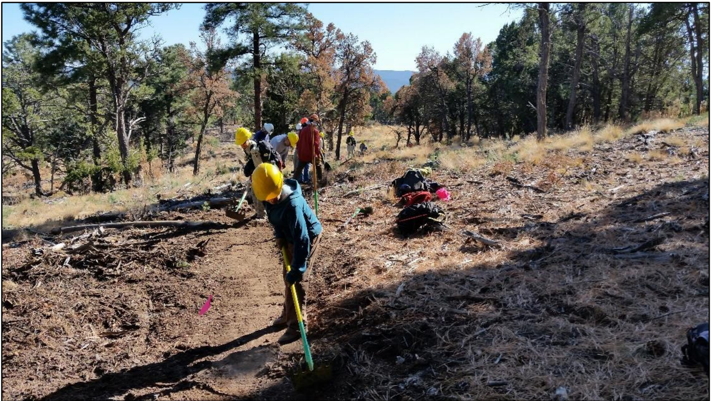
During: The crew picked up steam as they sensed the end of the line.
