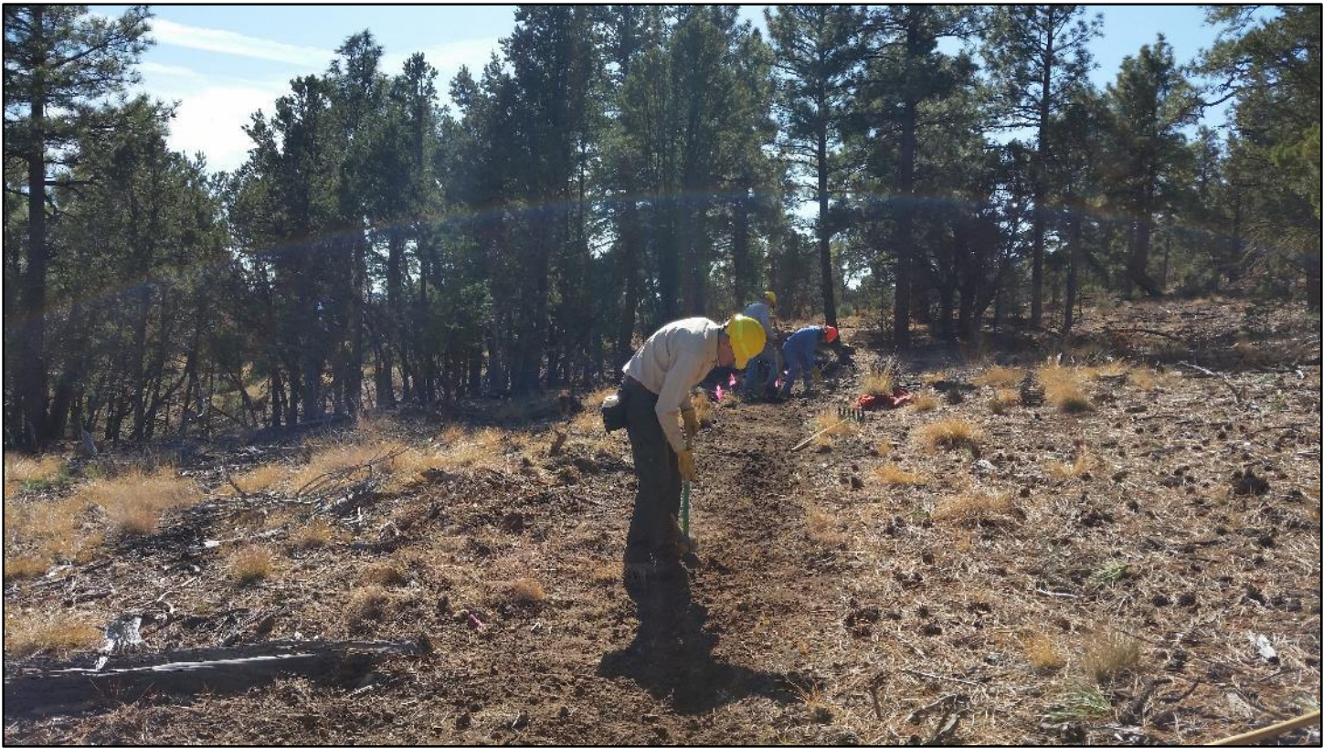
Leveling the tread is always the last step in a new section.
