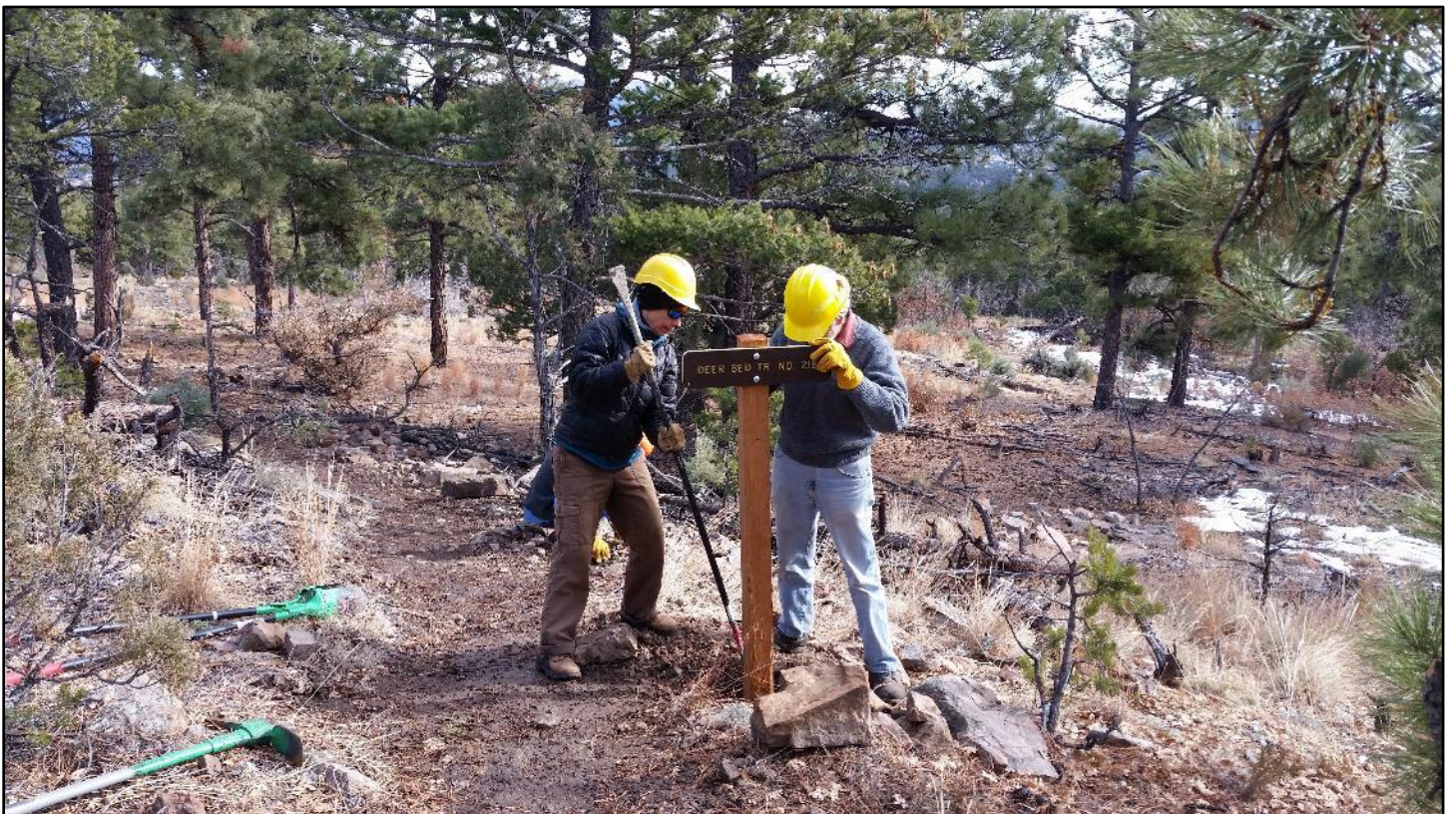
Pack it in. The wet soil and many rocks provided ideal materials to secure the sign.
