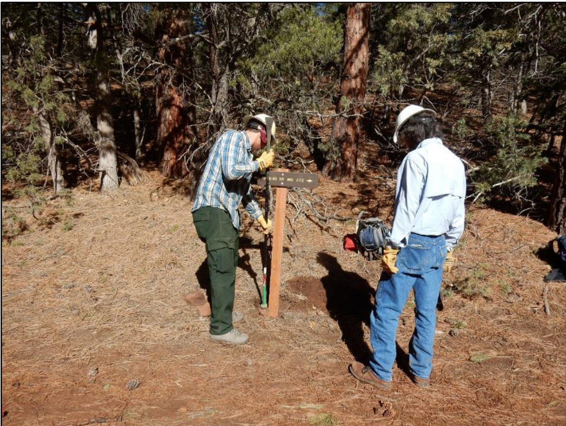
Packing many rocks in around the sign at the Valle/Armijo Trails junction.
